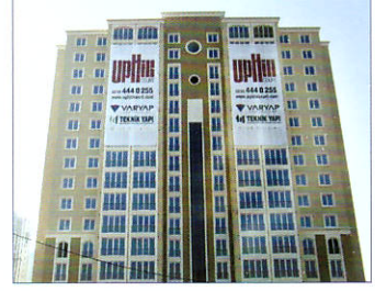
UPHILL COURT Ataşehir / İSTANBUL 1742 Konut
